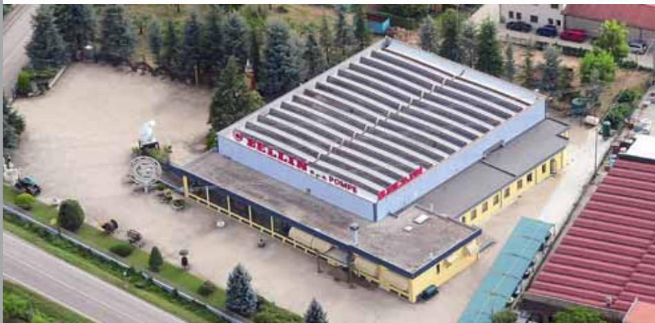
HEADQUARTERS - PRODUCTION UNIT 2
